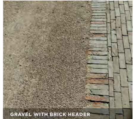
GRAVEL WITH BRICK HEADER
